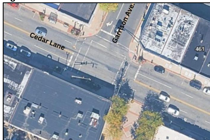
Fig. 6: Intersection of Cedar Lane and Garrison Ave.
