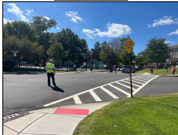
Fig. 9: High Visibility Crosswalk, "Slow School Zone" Sign
