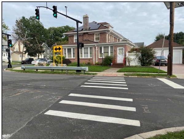
Figure 43: Crosswalk on Magie Avenue
